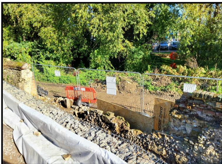
Collapsed section of Merton Priory precinct wall under repair
