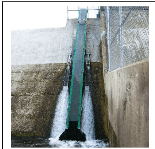
Figure 10 An Eel ladder in Canada - look how steep and high it goes
