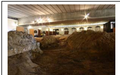
Figure 6 – a close up showing the depth of the trench
