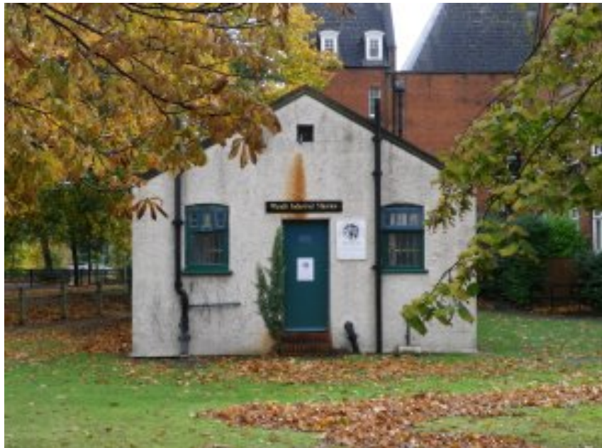
Figure 7 – the new rear signage...
